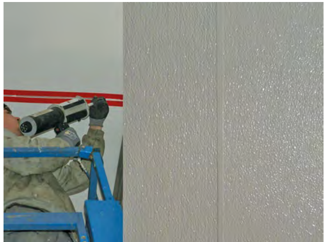
Figure 5. The HygiSeal seamless joint connection.
