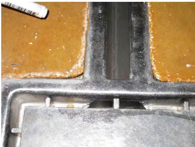
Figure 3. Sharp angles and a lack of flexible sealant where the resin floor meets the channel create crevices that can retain contaminated water.
