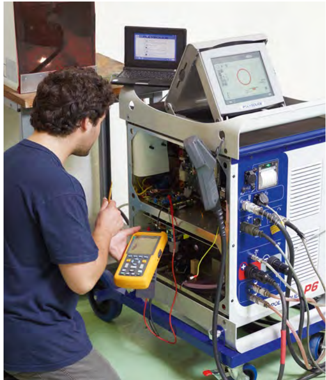
Figure 2. Checking and calibration a printed circuit board during, and after a maintenance operation on a power source.
