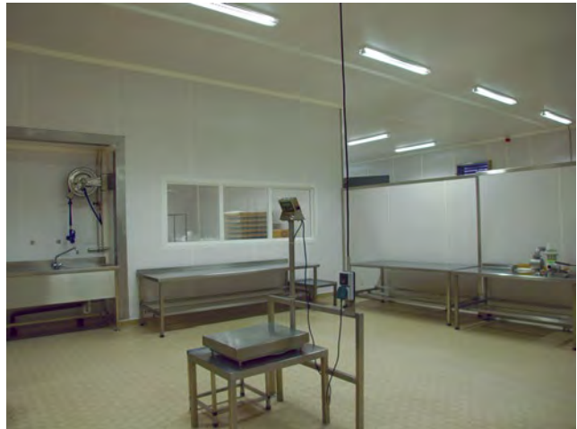
Figure 4. Finished renovations of food production areas with FRP solutions.
