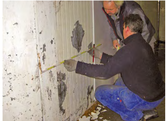
Figure 2. Installation of FRP on the damaged and corroded steel sandwich panels.
