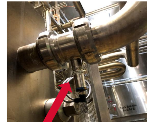
Point of Installation: In line(after pasteurizer)
